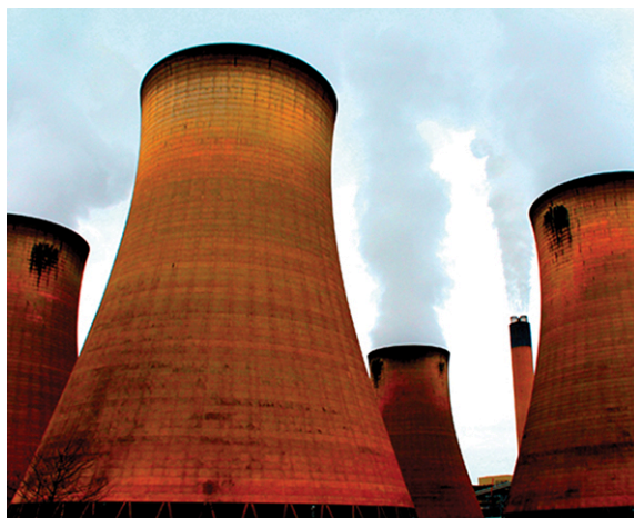
Figure 10 Cooling towers at the Drax power station in North Yorkshire, United Kingdom (credit: Les Haines, Flickr)
